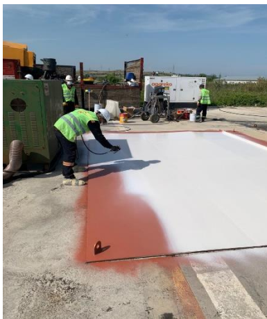
PUMMA application by airless sprayer.
