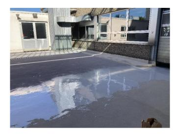
After priming the substrate with Plastifloor® 112 (dry substrate) or 118 (slightly wet substrate) the coating system will be applied in 1 or 2 layers. We recommend the 2 layer system when the substrate shows cracks and in harsh weather conditions like in northern Europe or North America.
